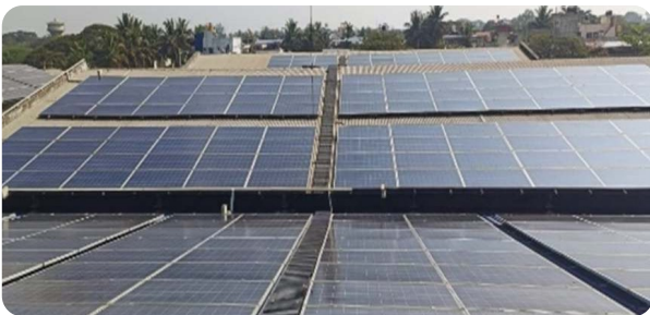
Image 1: Showing the Photovoltaic cells being installed on the roof of JRM to harness Solar Energy.
